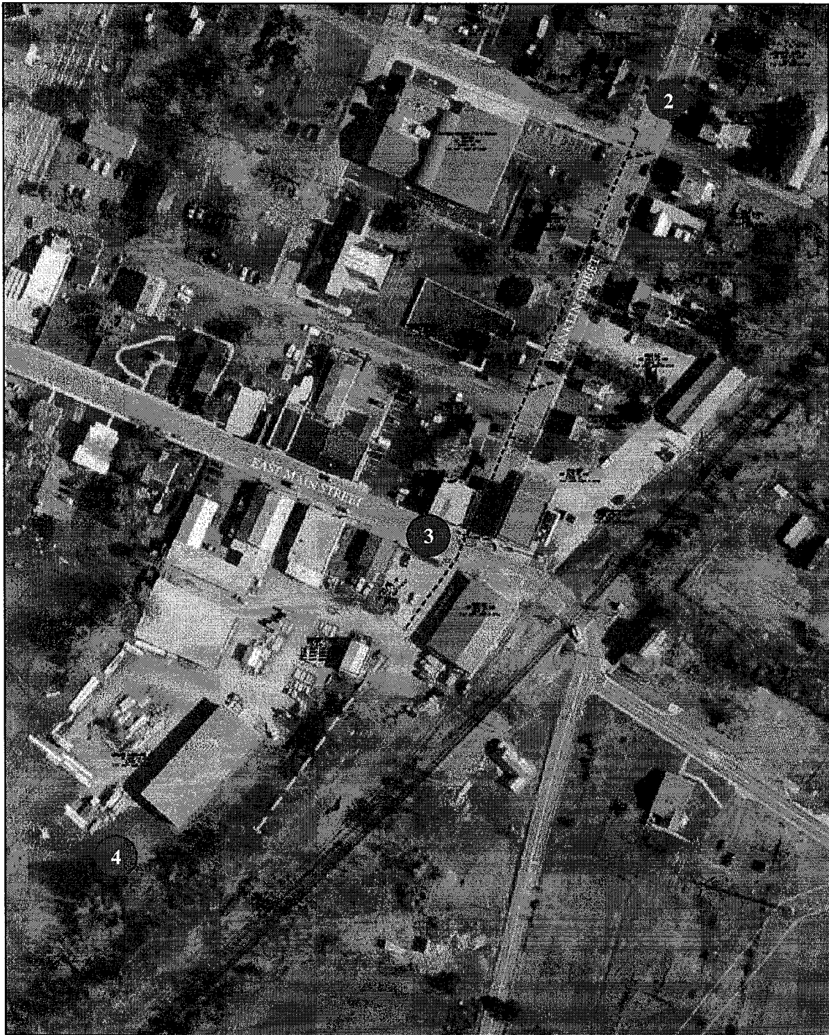
FIGURE 1.4: VDOT PLAN FOR FRANKLIN STREET FLOODING
